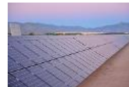
Solon UASP 3 Fixed PV 4.0 MW
