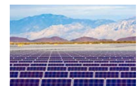
Picture Rocks Solar Fixed PV 20 MW
