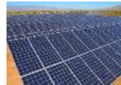
Solon Prairie Fire Fixed PV 4.0 MW
