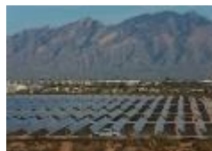
Valencia Solar Single Axis Tracking PV 10 MW
