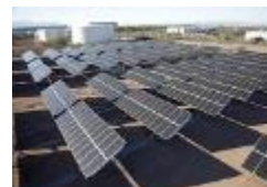
Solon UASTP 1 Single Axis Tracking PV 1.3 MW 500 kW of Lithium-Ion Battery Storage
