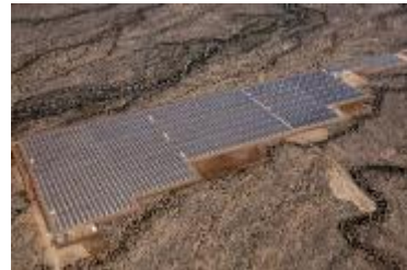
Black Mountain Solar Fixed PV 8.9 MW
