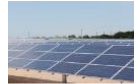
E.ON. Single Axis Tracking PV 4.8 MW
