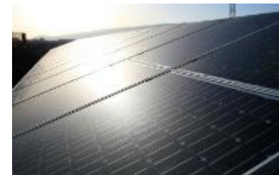
Red Horse Solar Fixed PV 30 MW
