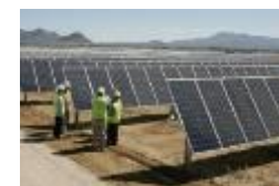
NRG Avra Valley Fixed PV 25 MW
