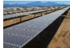
Avalon Fixed PV 28.3 MW
