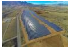
Fort Huachuca Fixed PV 13.6 MW
