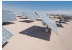
Amonix Dual Axis Concentrated PV 1.2 MW
