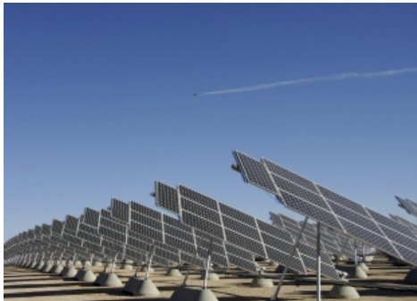
Single Axis Tracking Systems 45 MW
