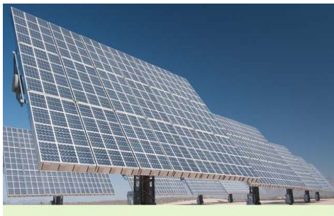
Concentrated PV 4 MW • U of A Science & Tech Park • Emcore
